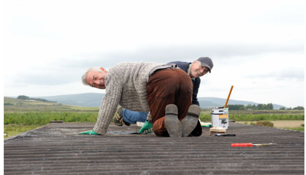
The clubhouse roof is once again weatherproof !
